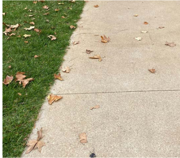
↑ INSITU CONCRETE (REFER OPTIONS FOR PERIMETER PATH)
