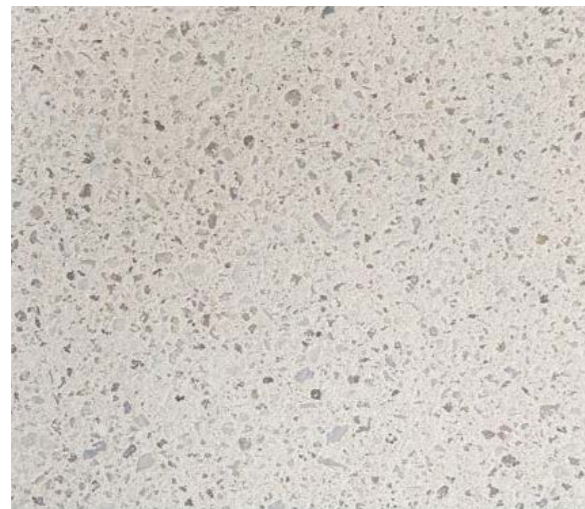
↑ NEW CONCRETE PATH
